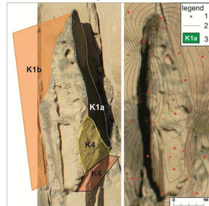
Fig. 4 – Rock pinnacle formed by four intersecting joint sets (no. 6 in fig. 2 and tab. 2): 1) point cloud; 2) contour line of the UAV-DTP (every 0.2 m); 3) joint set of the discontinuities surveyed on the slope (see fig. 3)
